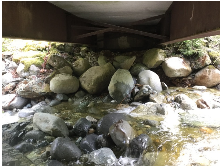
Right Bank Abutment when facing downstream
