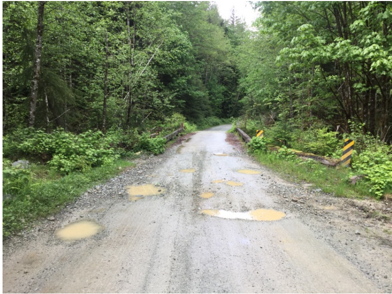
Approach from Right Bank when facing downstream
