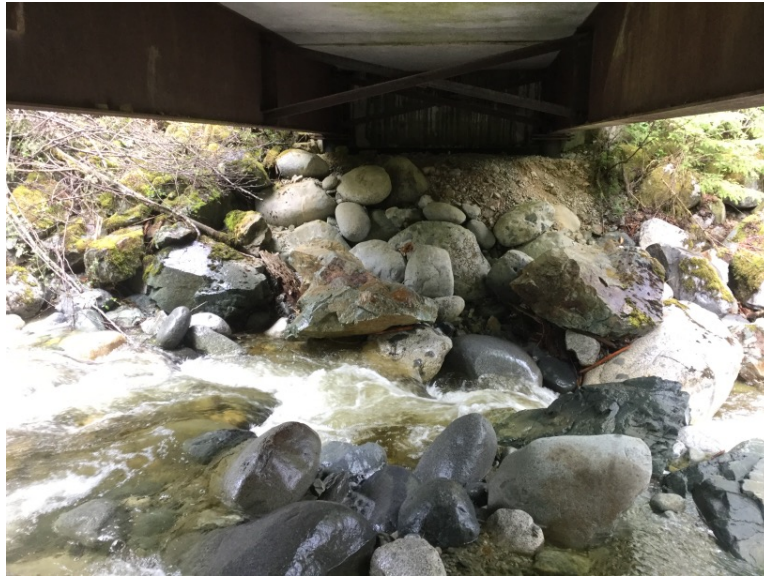
Left Bank Abutment when facing downstream
